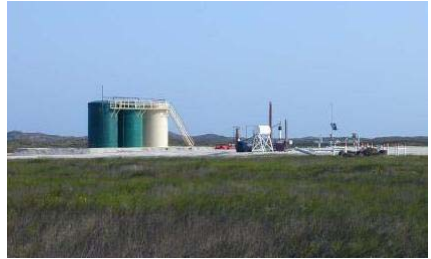
Surface facilities at La Playa, Padre Island
